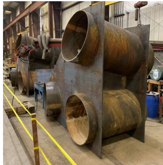
Figure 8 – Foundation Pile Nodes in Fabrication
