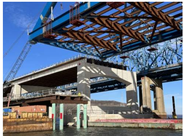
Figure 34 – Moving over Piers
