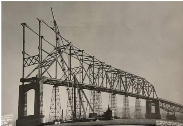
Figure 3 – Original Bridge Construction
