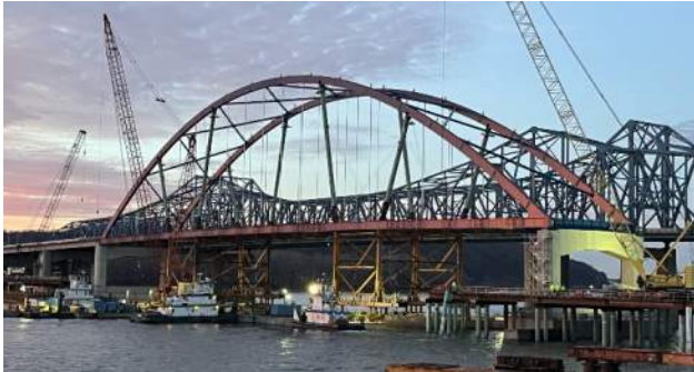
Figure 35 – Float-In Complete
