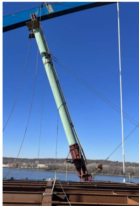
Figure 20 – Adjustable Arch Struts
