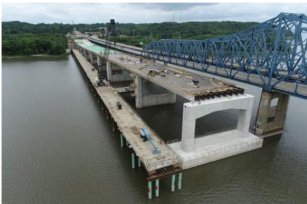
Figure 15 – Crane Trestle Structure
