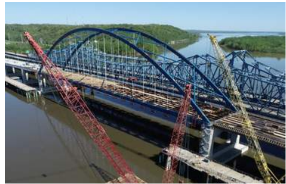
Figure 36 – Installation of Deck Forming System
