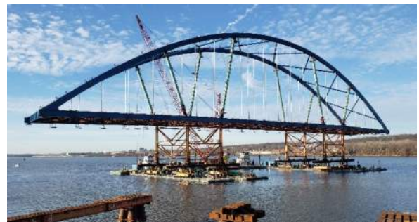
Figure 28 – Span during Float-In
