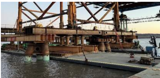
Figure 26 – Barge Grillage and Initial Setup
