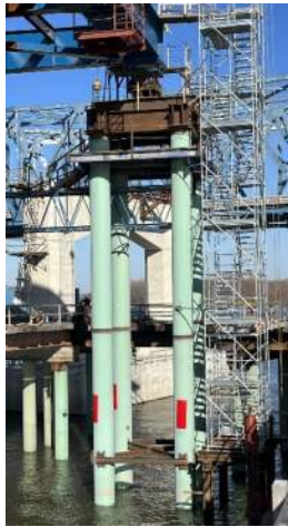
Figure 13 – Knuckle Falsework Structures
