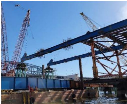
Figure 18 – Floor System Erection
