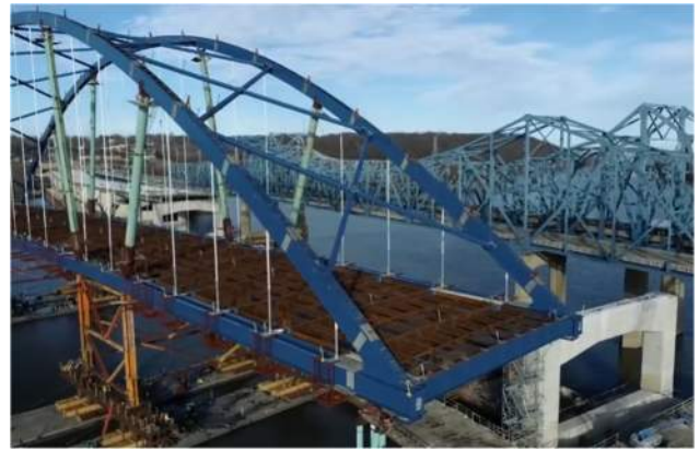
Figure 32 – Preparing to Move Over Piers
