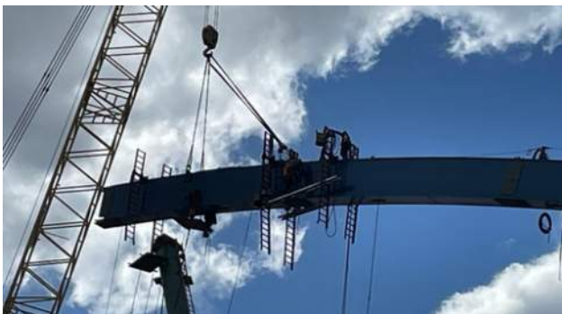
Figure 22 – Arch Segment Lifting and Rigging
