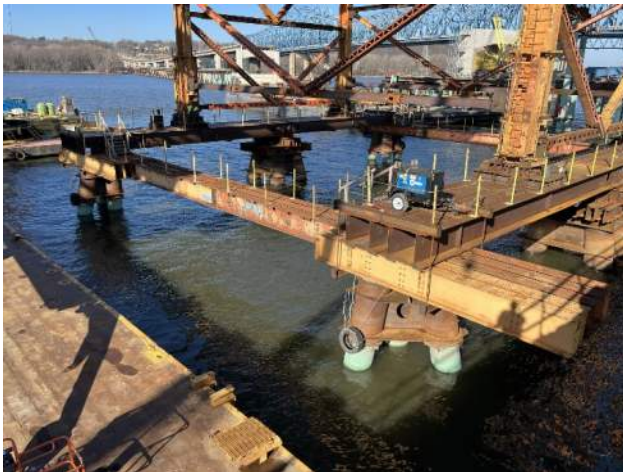
Figure 10 – Main Support Falsework Foundation
