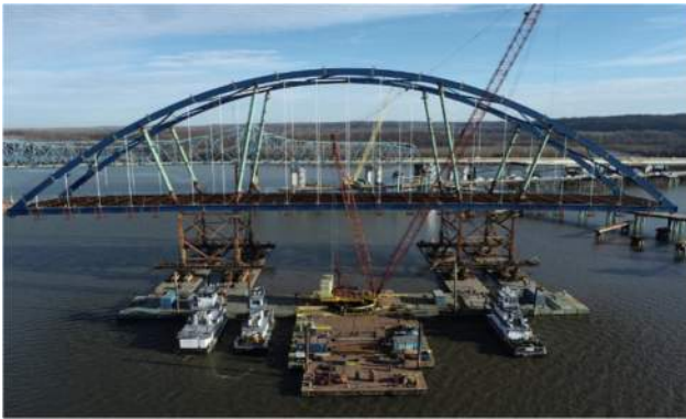
Figure 29 – Span during Float-In
