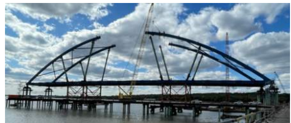
Figure 25 – Arch Erection
