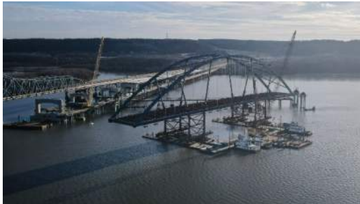
Figure 30 – Span Moved Upstream
