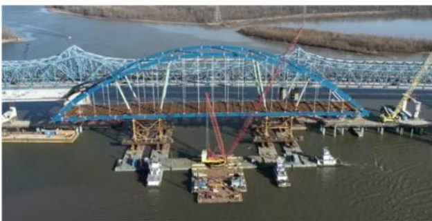
Figure 31 –Float-In Nearing Final Location
