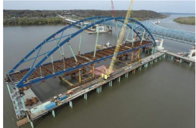
Figure 16 – Crane Trestle for Arch Span Erection
