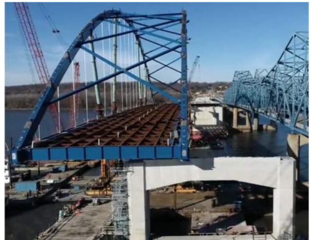
Figure 33 – Moving over Piers
