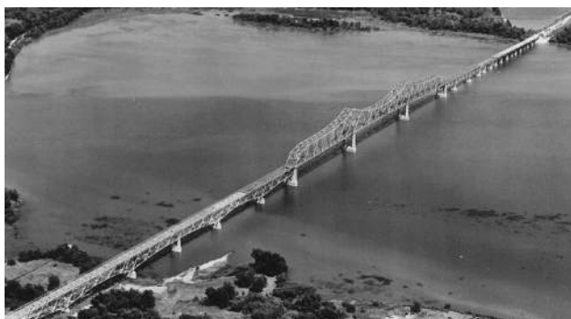
Figure 4 – Original Bridge Construction
