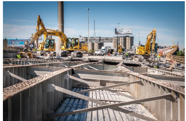
Figure 14 – Deck Removal Operation
