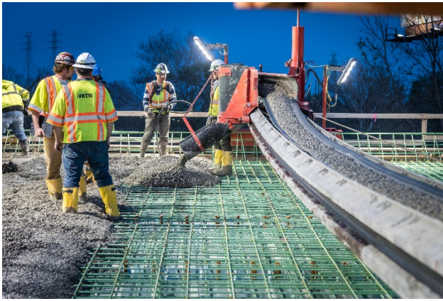
Figure 21 – New Deck Construction
