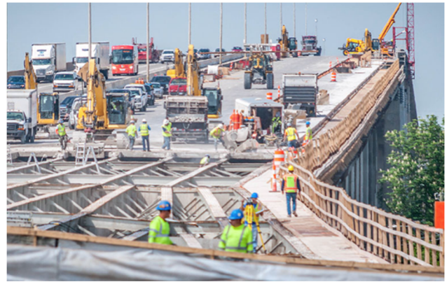
Figure 13 – Deck Removal Operation
