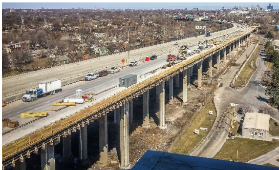
Figure 11 – Equipment on Deck
