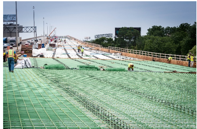
Figure 19 – New Deck Construction
