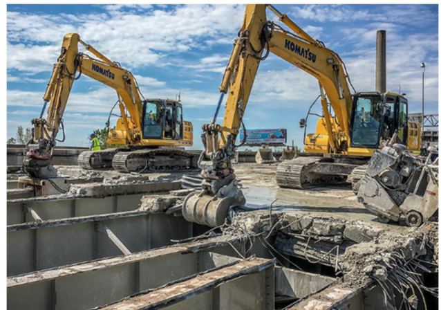
Figure 15 – Deck Removal Operation
