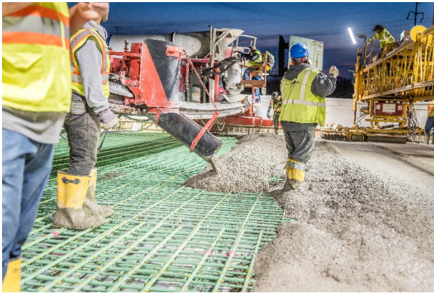
Figure 22 – New Deck Construction
