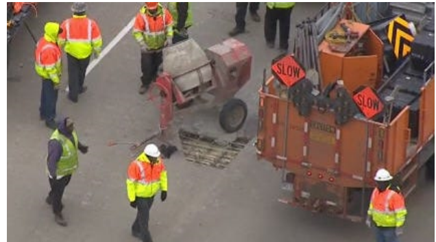
Figure 6 – Deck Repairs Prior to Project
