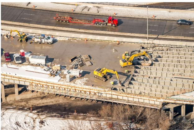
Figure 12 – Equipment during Deck Removal
