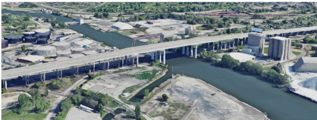
Figure 4 – Zone of Bridge over Rouge River
