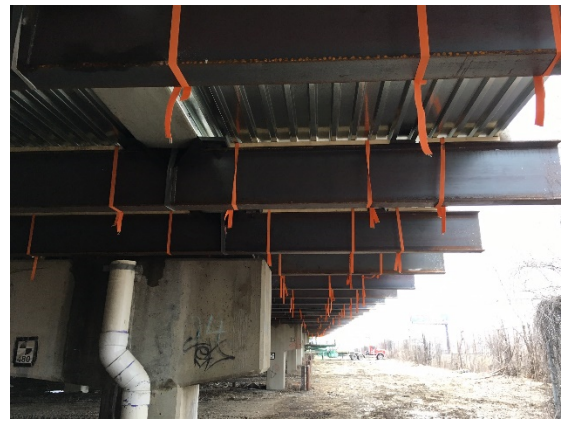
Figure 18 – Fascia Overhang System
