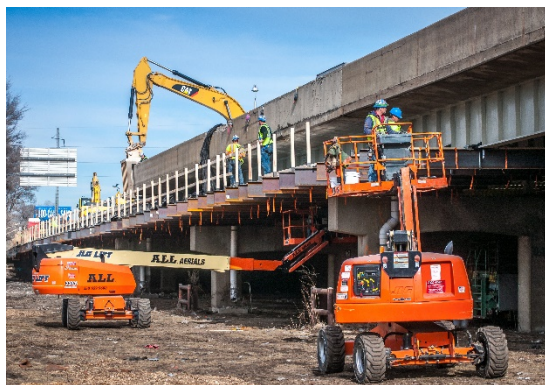
Figure 17 – Fascia Overhang System
