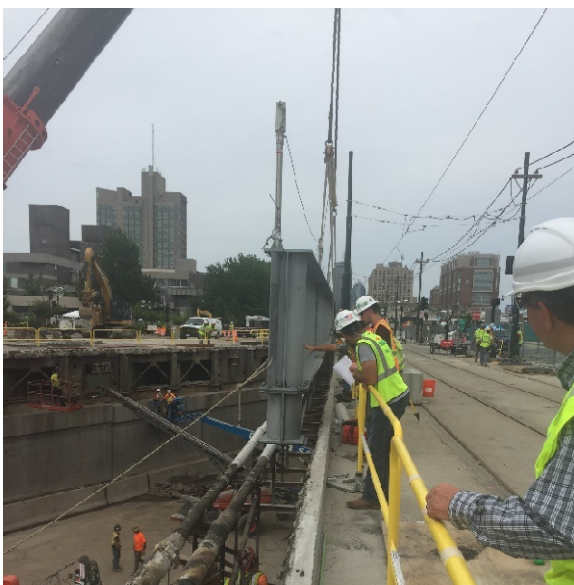
Photo 17 - New Girder Set Around Live KV Lines during Outage 2
