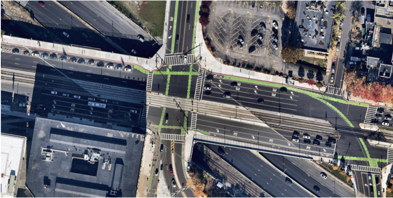
Photo 1 – Plan view of Intersection Between Commonwealth Avenue Bridge / I-90 / MBTA Commuter Rail
