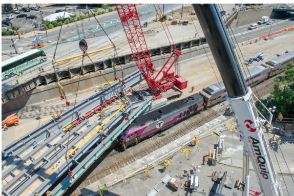
Photo 11- Span 1 Girders Set as Singles
