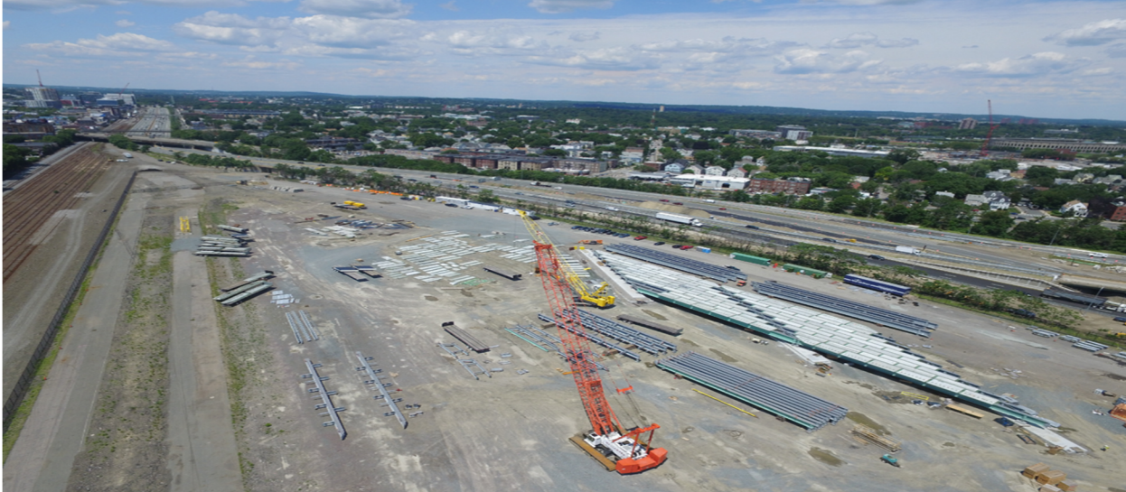
Photo 6 – Pre-Assembled Bridge in Staging Yard
