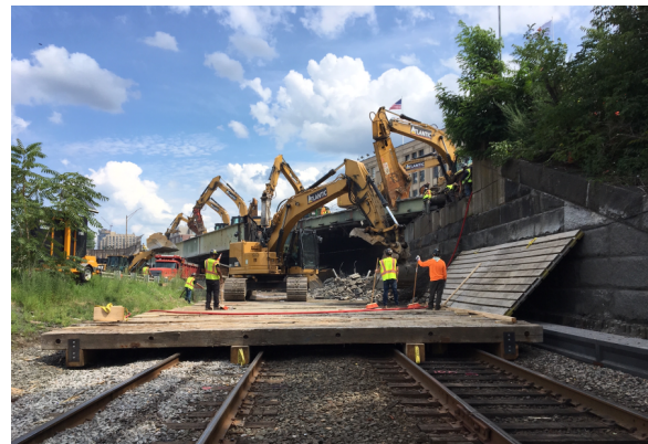
Photo 15 – Track Protection over MBTA Commuter Rail Line
