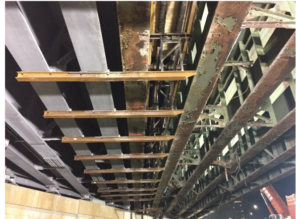
Photo 4 – 115kV Temporary Supports After Deck Removal
