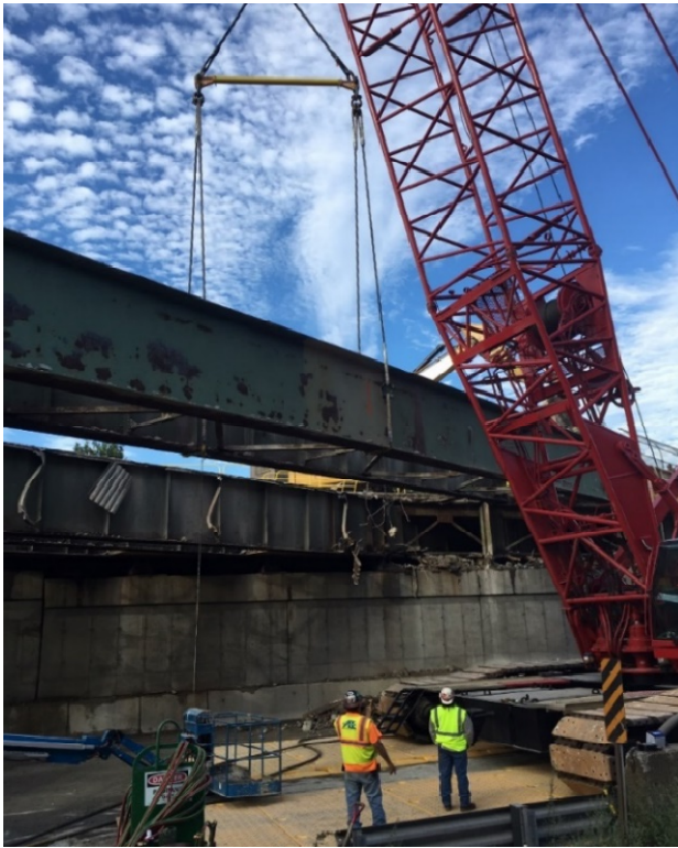
Photo 10 - Removal of Existing Span 2 Girders as Pairs during the First Outage
