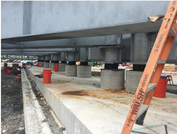
Photo 5 - Temporary Footings and Pedestals at Staging Yard
