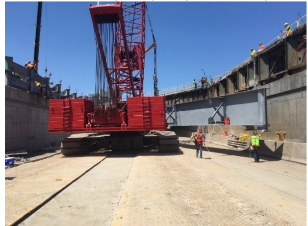
Photo 12 – 400 Ton Manitowoc Crawler Crane in I-90 during the First Outage
