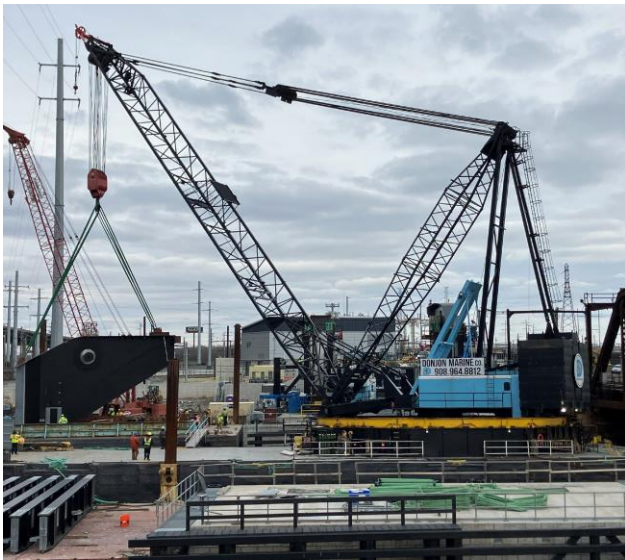
Figure 9 – Heavy Lift Crane Barge Erecting Heel Girder
