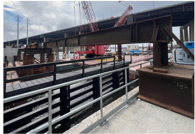
Figure 11 – Temporary Pile-Driven Support Tower
