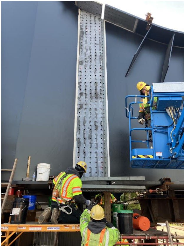
Figure 12 – Heel to Main Girder Field Splice
