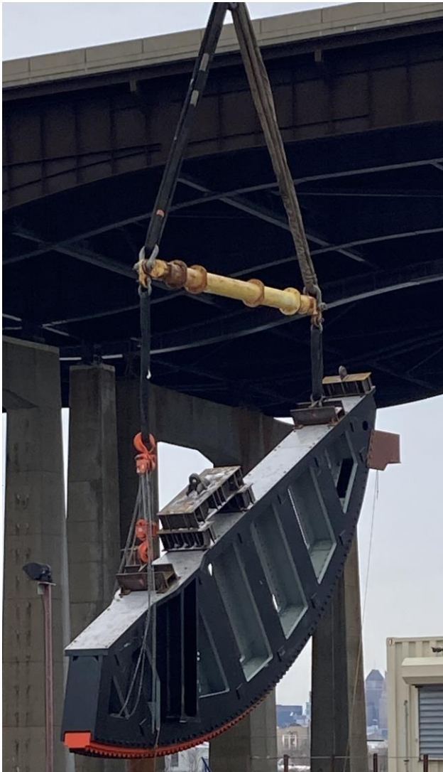
Figure 6 – Gear Rack Lifting Assemblies (vertical lifting for final erection shown)
