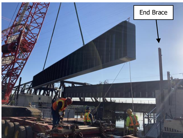
Figure 4 – Span 5 Girder Erection
