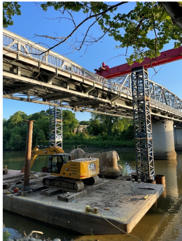
IMG 4 - Spans Supported by Falsework
