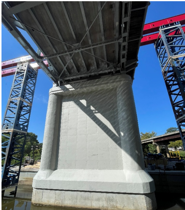
IMG 3 - New Pier
