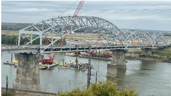
Figure 2 - Main River Span Unit 4
