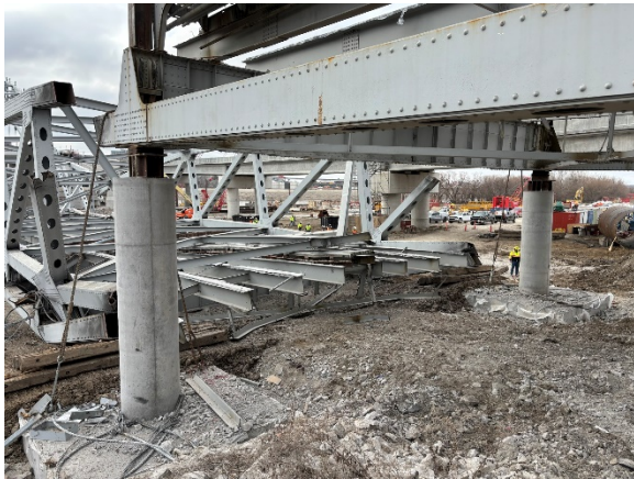
Figure 11 - Temporary Falsework Bent
