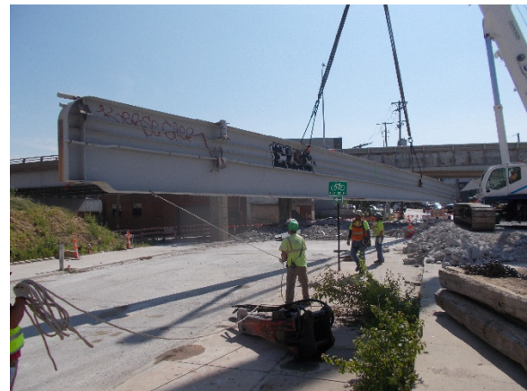
Figure 18 - Unit 1 Girder Removal
