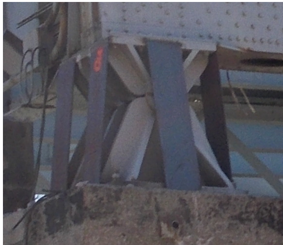
Figure 13 - Pier 4 Uplift Restraint
