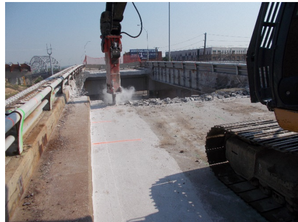
Figure 16 - Unit 1 Deck Removal
