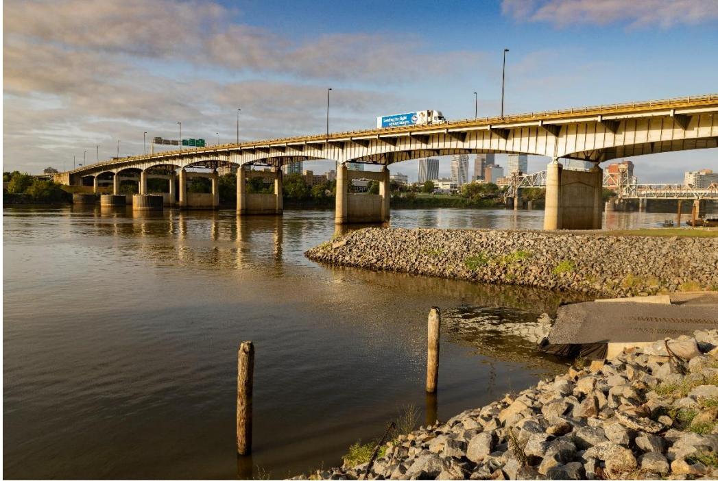
30 Crossing construction, Little Rock, Arkansas. September 26, 2020. ©David Hoge
