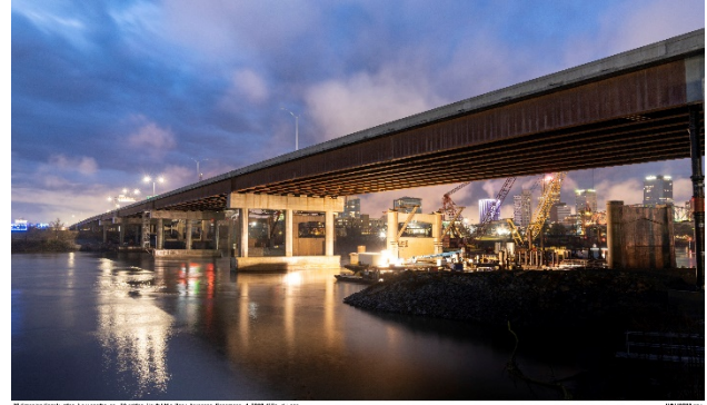
Figure 20 - New EB I-30 Bridge
