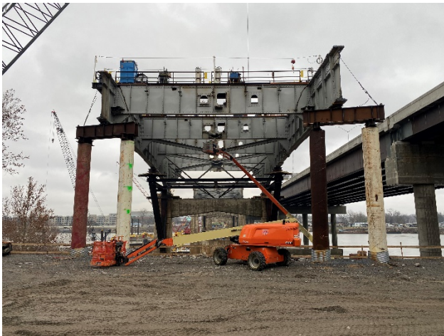
Figure 13 - Falsework Towers
