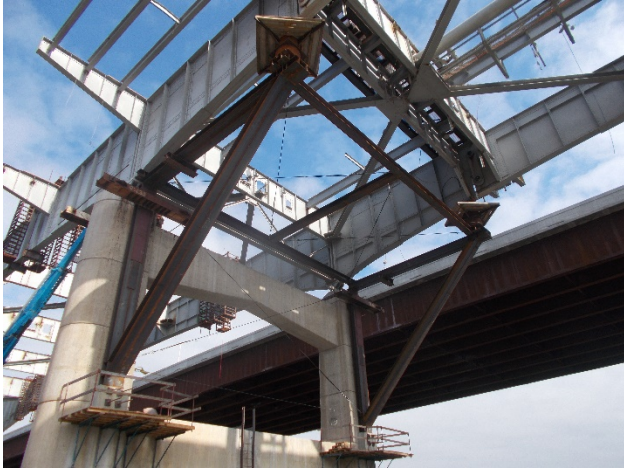
Figure 7 - Pier Bracket
