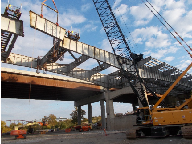
Figure 17 - Individual Girder Pick
