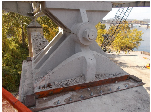
Figure 18 - Longitudinal Bearing Restraint
