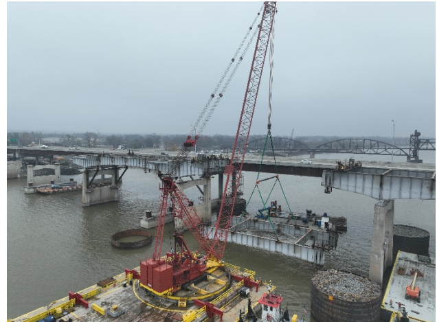
Figure 15 - Paired Girder Pick
