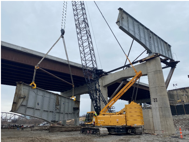
Figure 19 - Final Girder Brace
