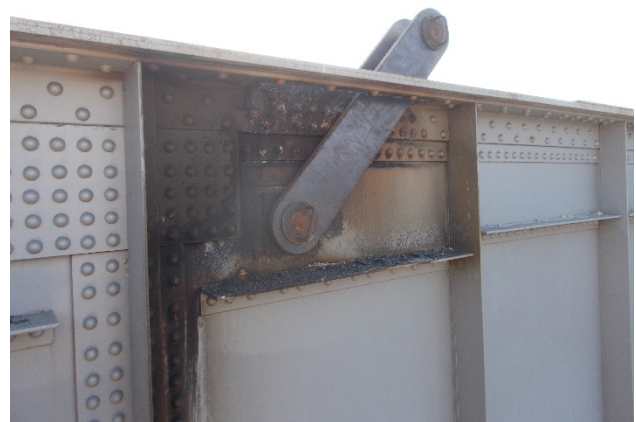
Figure 16 - Custom Lifting Lug
