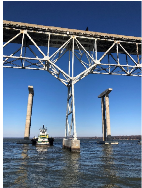
Figure 2 - View of 2D Plane Pier and Rhomboid Region
