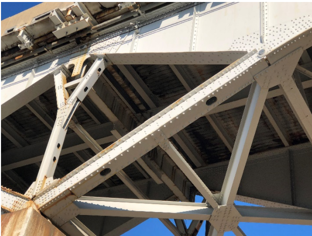
Figure 10 - Girder Span Pier Framing
