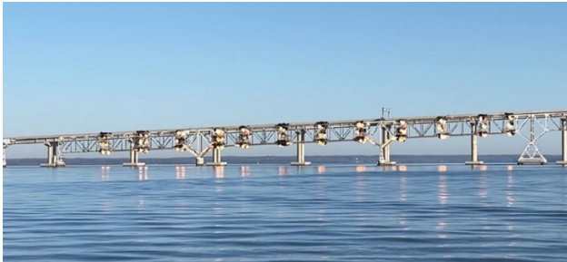
Figure 17 - Deck Truss Explosive Demolition
