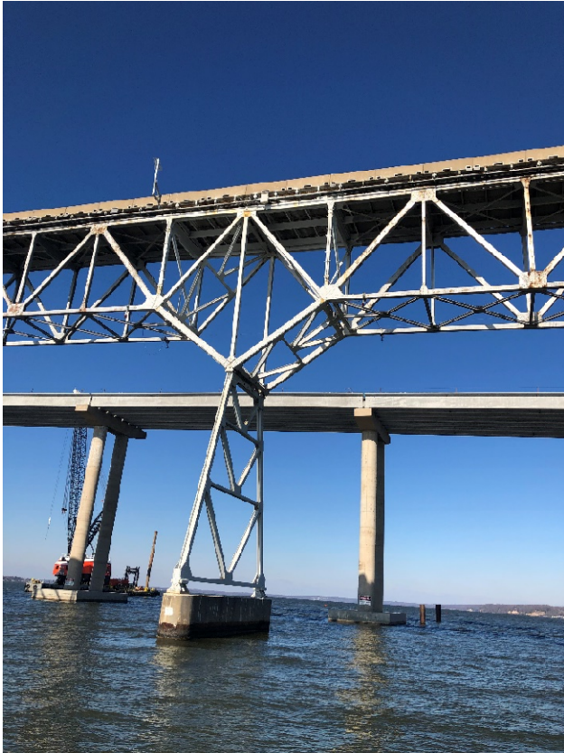
Figure 15 – Deck Truss Span Pier Framing
