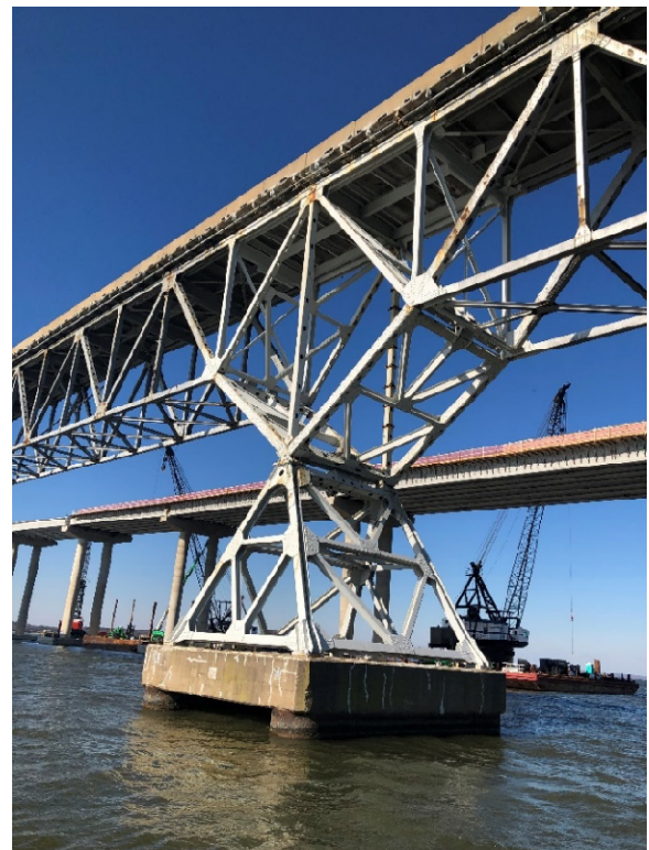
Figure 3 - View of Fixed Pier Tower
