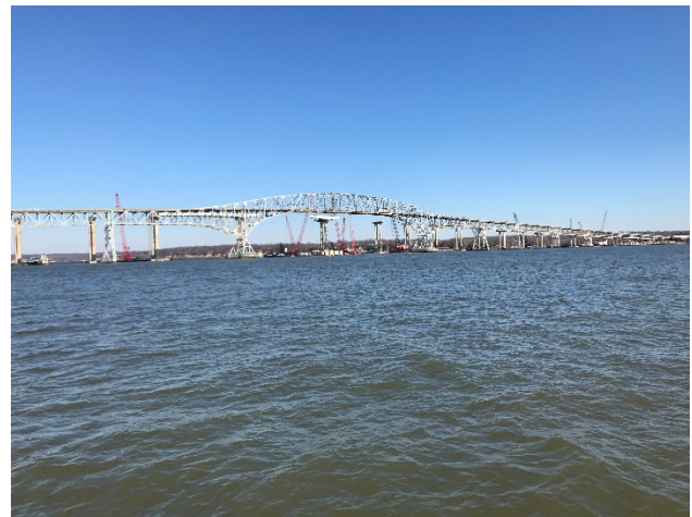
Figure 1 - Main Suspended Span and Anchor Spans
