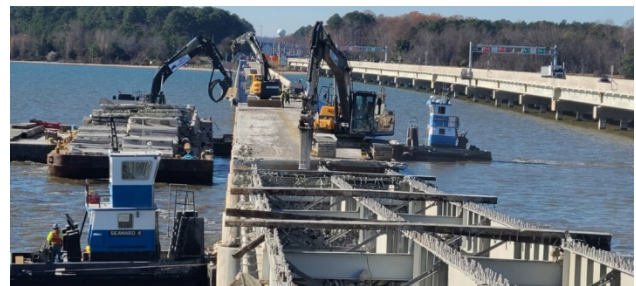
Figure 8 - Trestle Span Demolition
