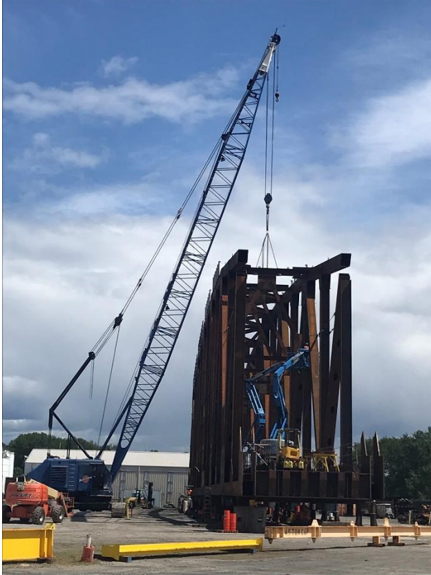
Figure 3 - Truss Assembly
