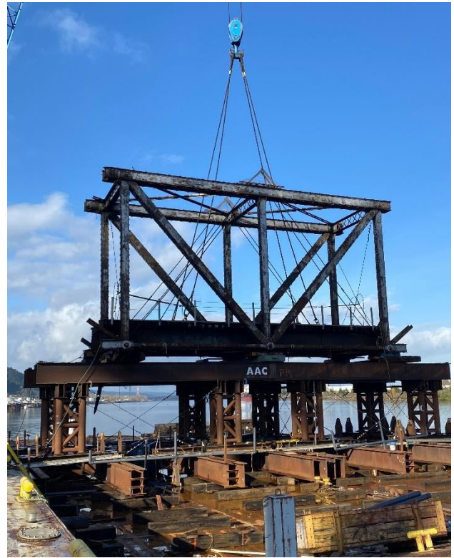
Figure 12 - Existing Truss Demolition
