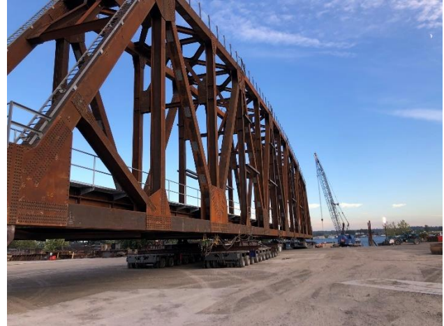
Figure 4 - Truss Roll On
