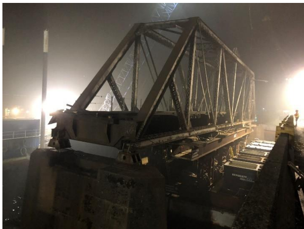
Figure 8 - Existing Truss Removal
