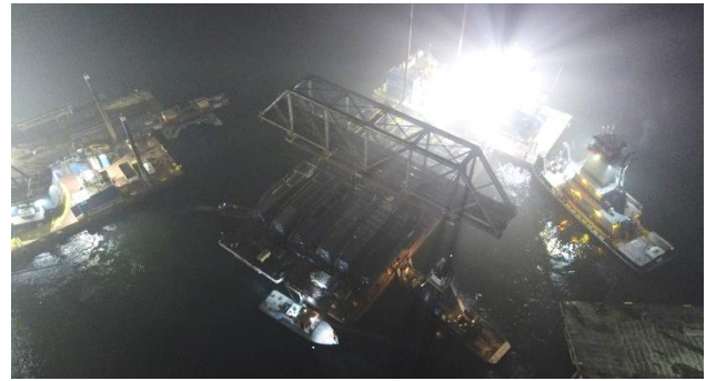
Figure 9 - Existing Truss Removal
