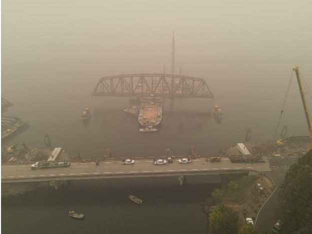
Figure 10 - New Truss Float In
