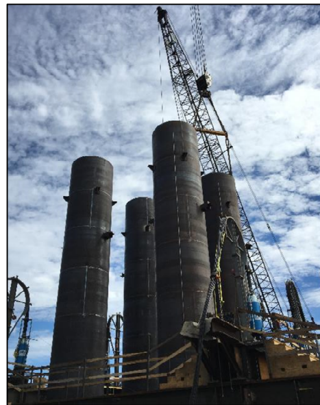
Photo 12 - First Lift of Casing Installed, Ready to Lower
