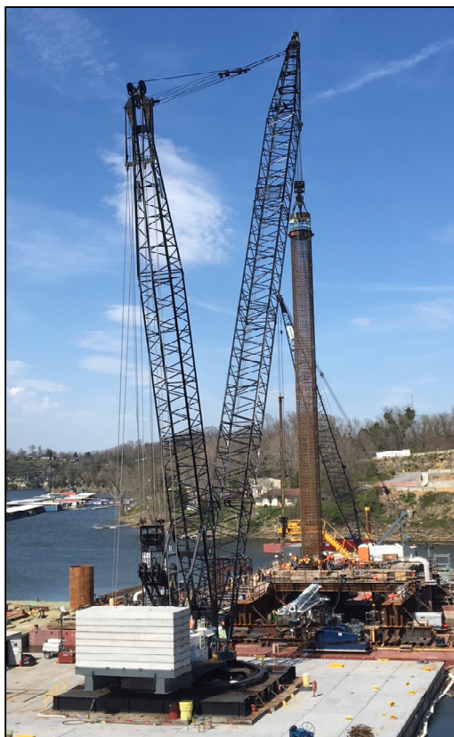
Photo 15 - 4100 Ringer Setting Rebar Cage
