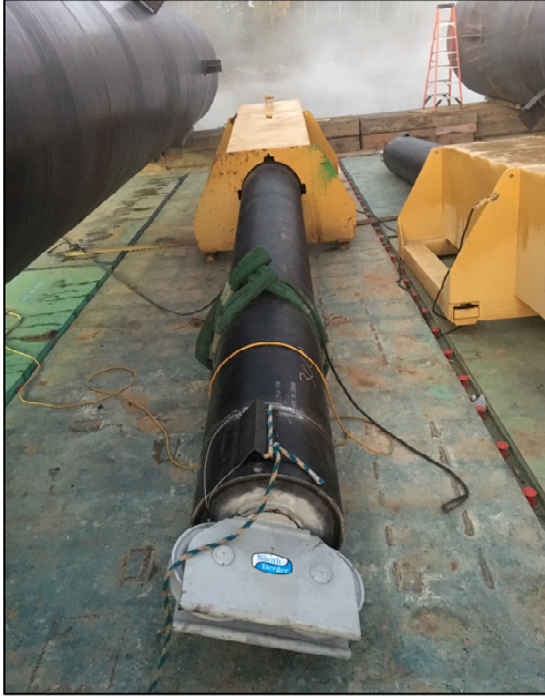
Photo 8 – 20-ft downrigger used to anchor the barge below water level to avoid boat traffic
