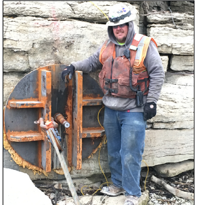
Photo 7 - Rock anchor used for barge horizontal alignment
