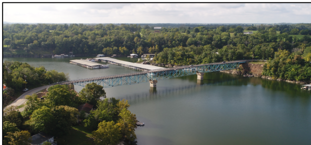
Photo 1 – Existing Truss Structure
