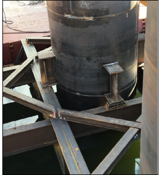
Photo 11 - Lower Lift of Casing Connected to Lowering Tray
