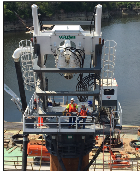
Photo 14 - Buma RCD Ready to Insert Drill String
