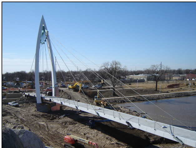
Fig. 3 – Arkansas River Bridge
