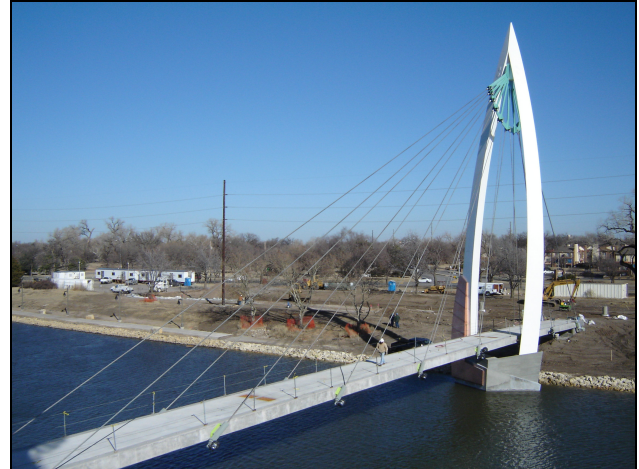
Fig. 4 – Little Arkansas River Bridge
