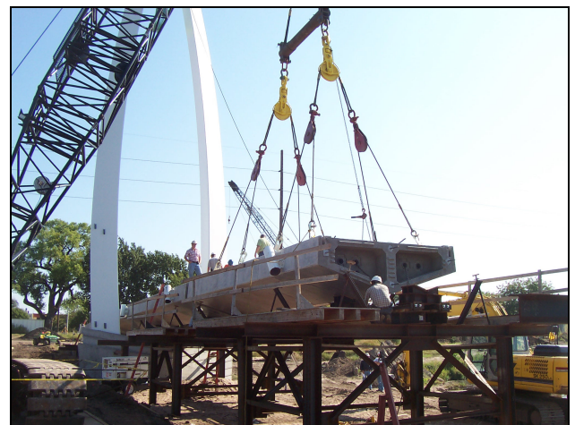
Fig. 12 – Deck Segment & Falsework Structures
