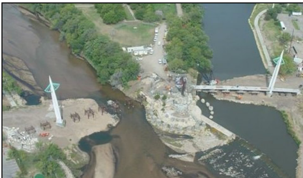
Fig. 1 – Bridge Construction Site
