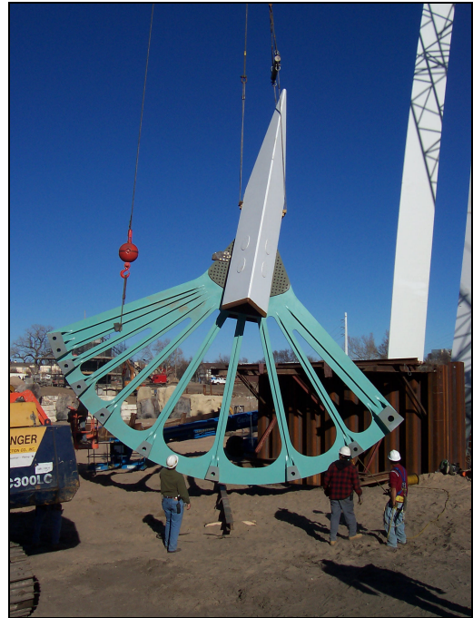
Fig. 8 – Upper Cable Anchorage
