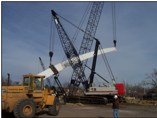
Fig. 7 – Tower Leg Crane Pick
