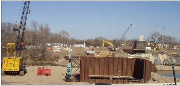
Fig. 6 – Typical Cofferdam
