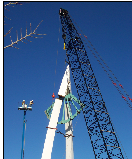
Fig. 9 – Upper Tower Crane Pick
