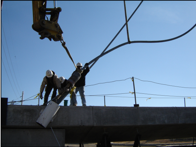
Fig. 15 – Typical Cable Installation
